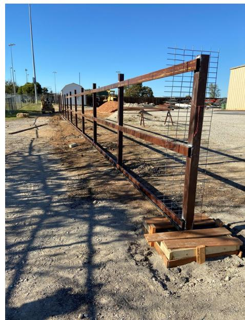
The new fence construction was somewhat time consuming due to the building of the metal cage columns that would be filled with decorative rock. The rock cages incase the steel posts on each side of the gate and corners. This was the first phase of the fencing project which will be continued soon.
